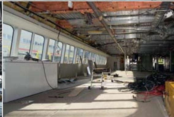
existing tier two passenger accommodation aft of frame 17. This module needed to accommodate approximately 300 passengers in a spacious 'airy' environment, with both bar and basic galley facilities, whilst seamlessly integrating with the rest of the vessel.
